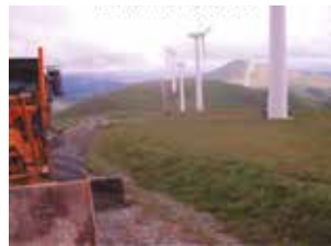
Access road maintenance
