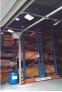
Digital Warehouse: RFID antennas for monitoring warehouse inputs and outputs.
