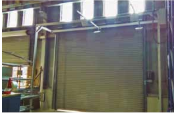
Digital Warehouse: RFID antennas for monitoring warehouse inputs and outputs.
